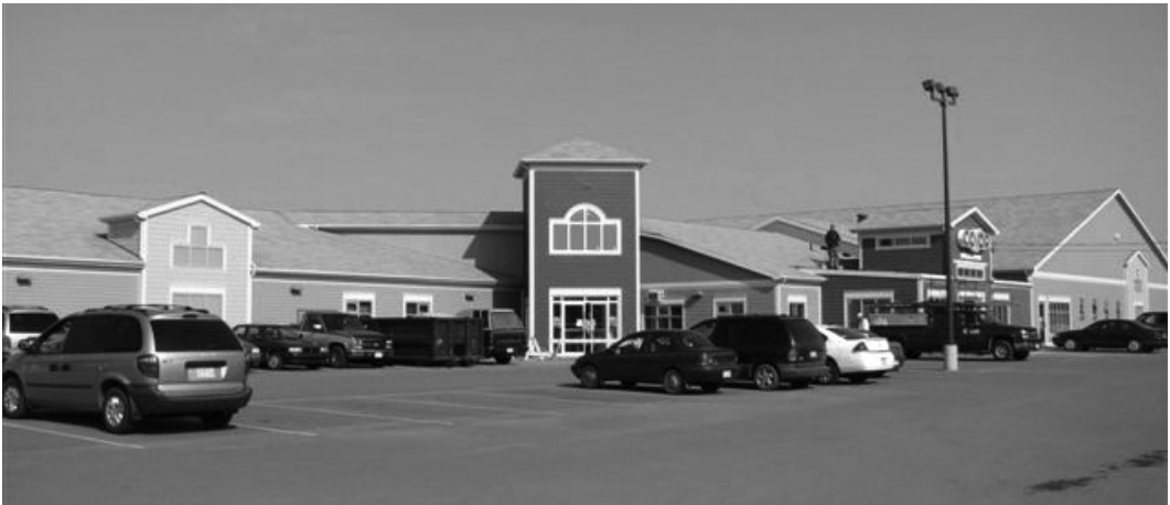
After the renovations.
